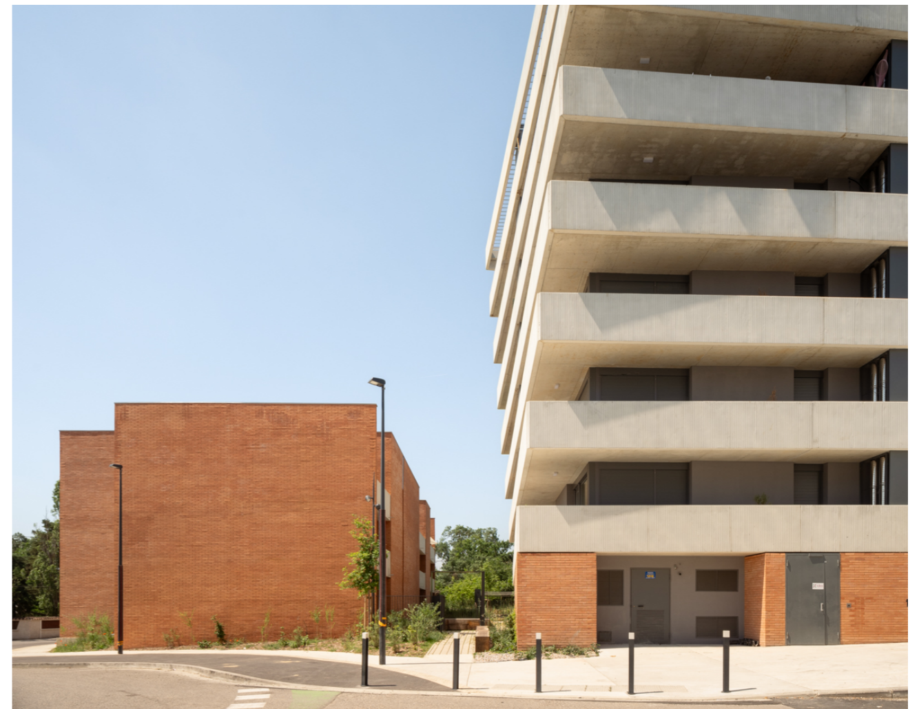
Architectures sans fenêtre. Architecture without windows.
